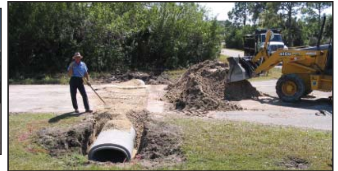
Pipe Replacement - Bryson Rd.
